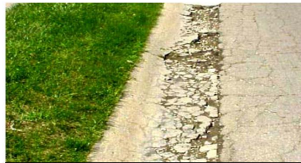
EXAMPLE: Exposed aggregate
