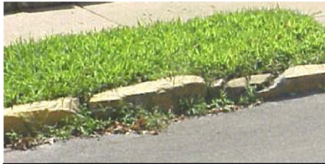
EXAMPLE: Settlement / Vertical Offset
