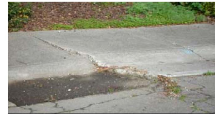
EXAMPLE: Asphalt repairs
